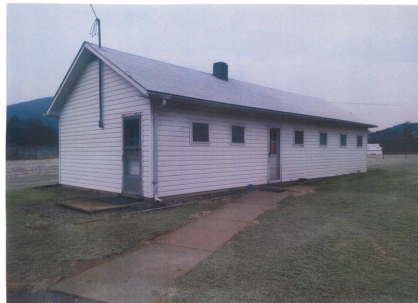
PICTURE OF BUILDING (SOUTH SIDE)
