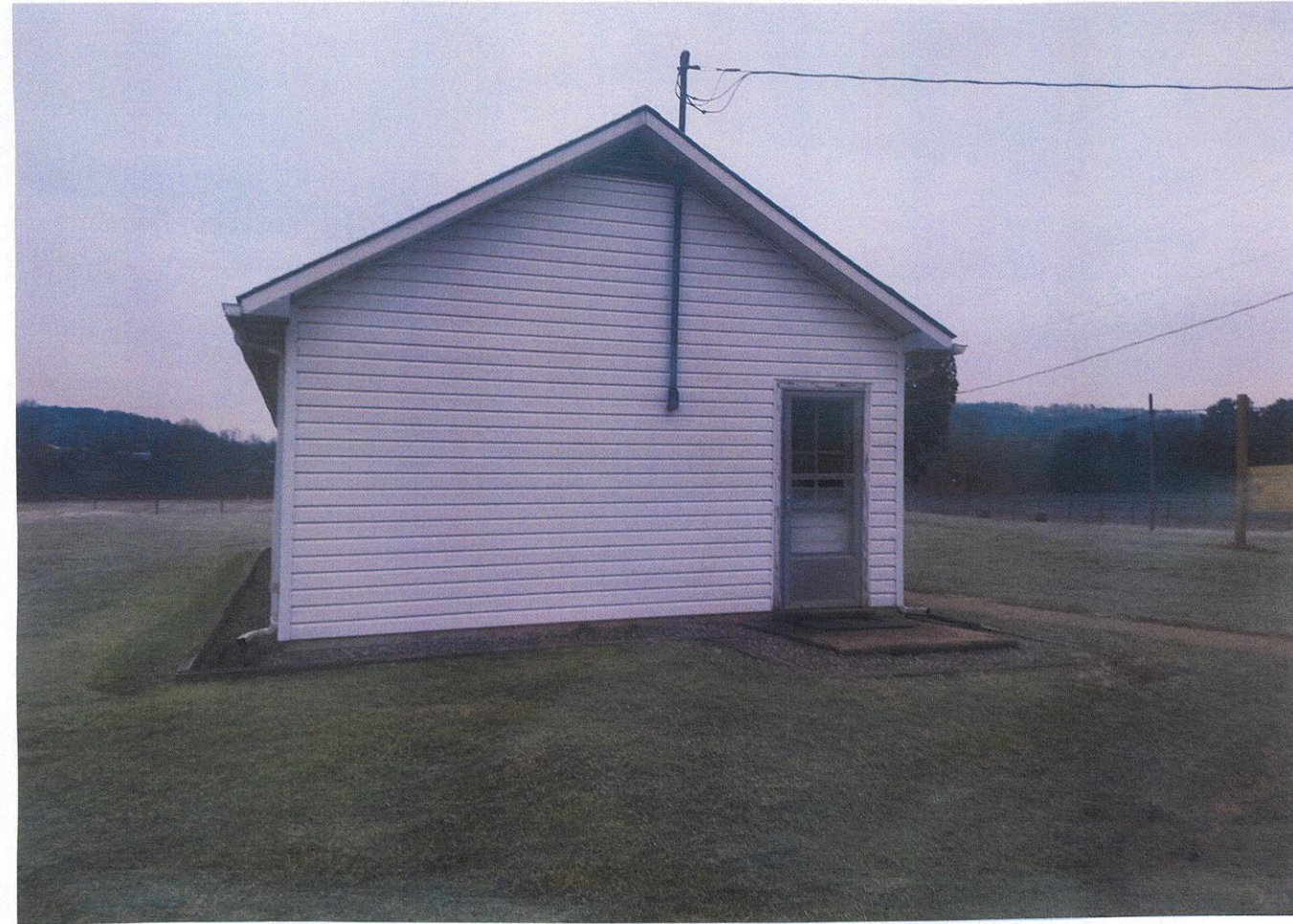
PICTURE OF BUILDING (WEST SIDE)
